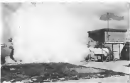
Fall cloud of steam during start. The airframe test installation appears to be heated and does discharge the exhaust pipe of a rocket or small jet engine test cell.
